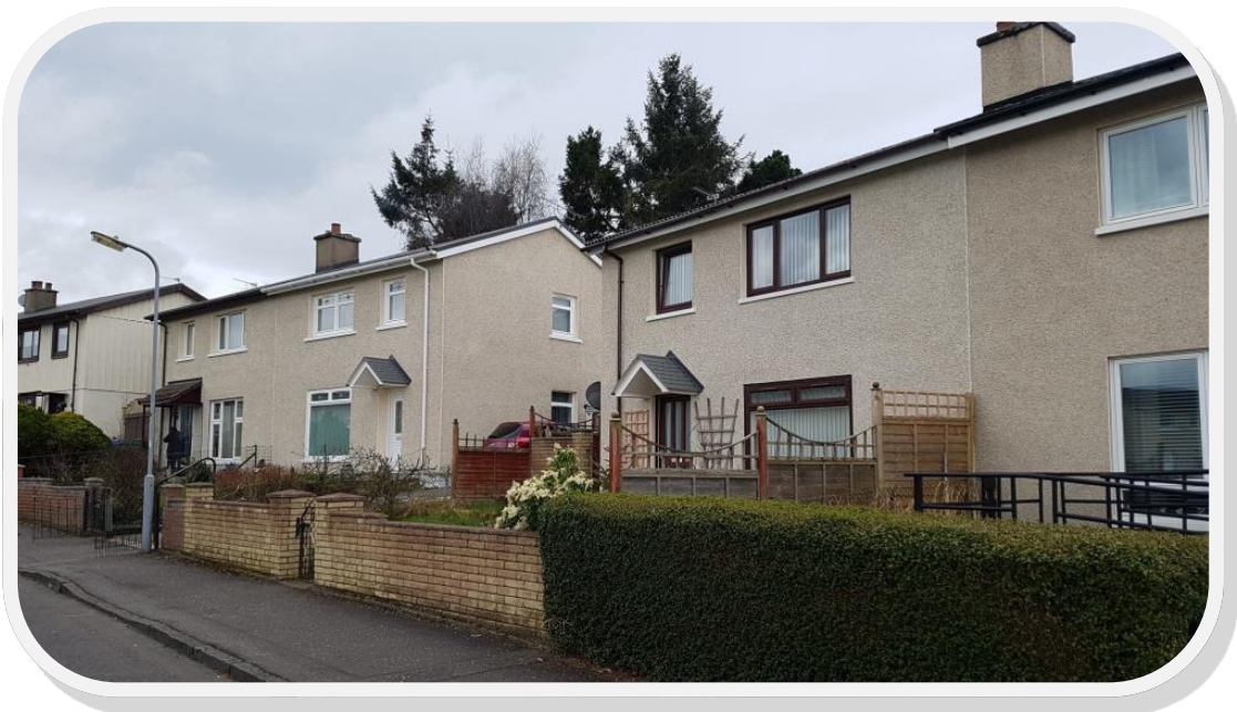
Fig 8. Completed houses in Forehill, Ayr
