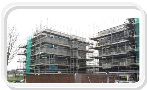
Fig 1. Insulation boards being fixed to all levels of flats.
